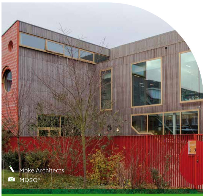
Public Elementary School "IKC" photo taken 5 years after installation - (320 m 2 ) Amsterdam, The Netherlands
