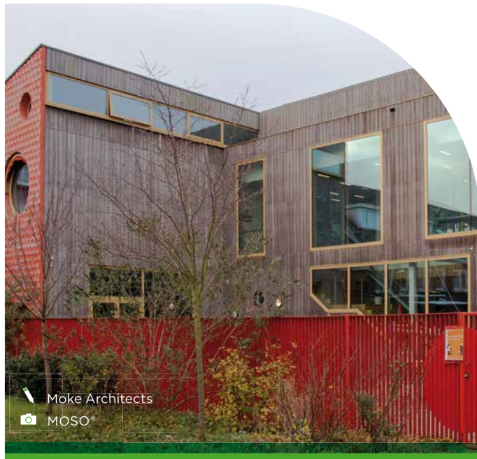
Public Elementary School "IKC" photo taken 5 years after installation - (320 m 2 ) Amsterdam, The Netherlands
